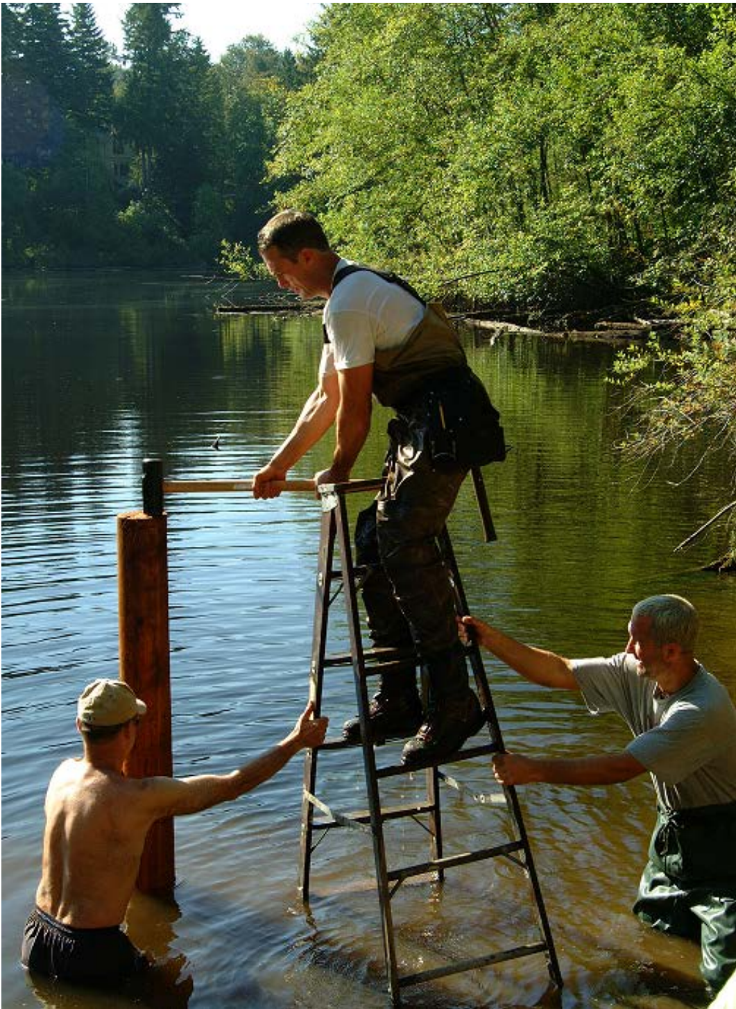
Using a step ladder to pound the corner posts into the substrate with a sledge hammer.
