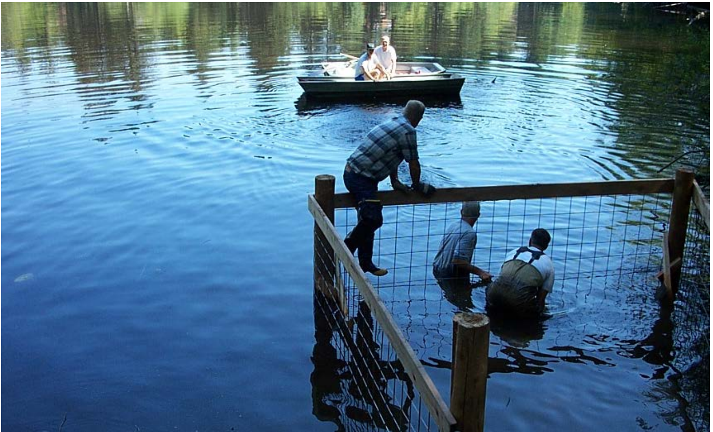
The pipe and round fence are placed on the bottom.
