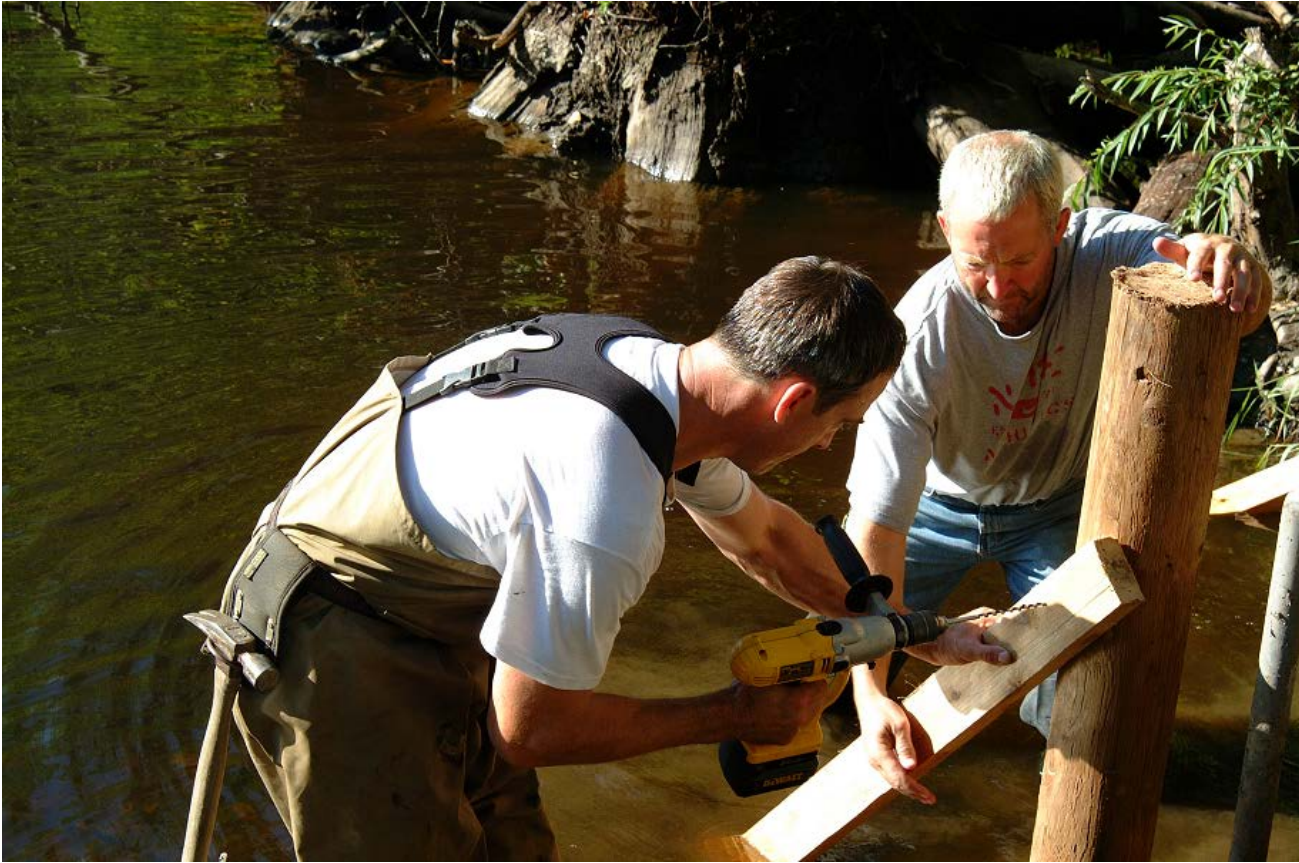
The receiver fence is installed at the mouth of the fish ladder or culvert mouth.
