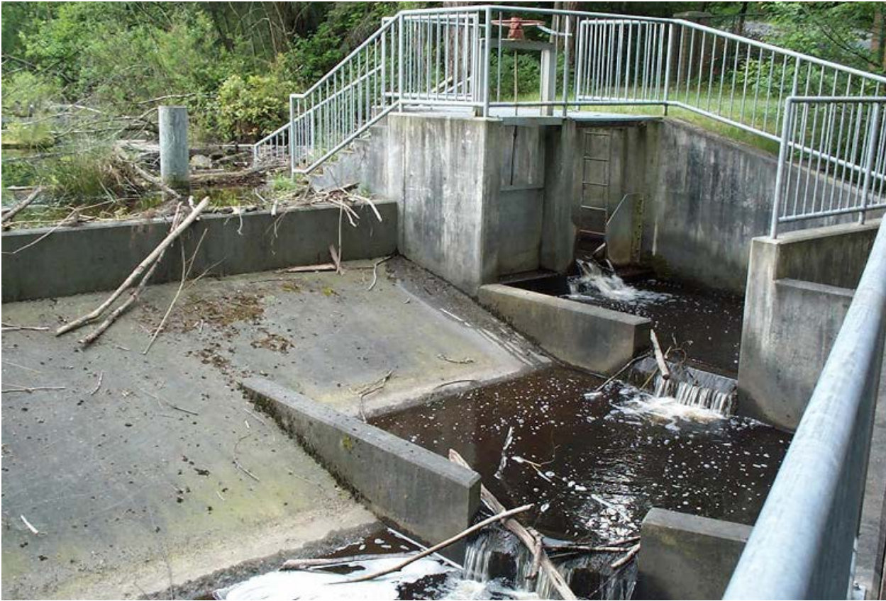
The upstream end of the fish ladder/outlet control structure
