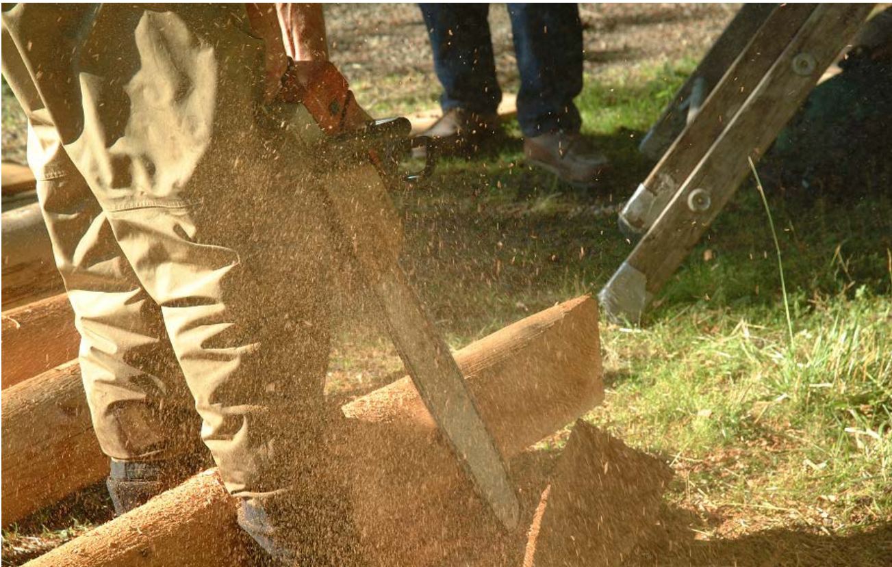
Cutting points on the corner posts makes it easier to pound them into the substrate.
