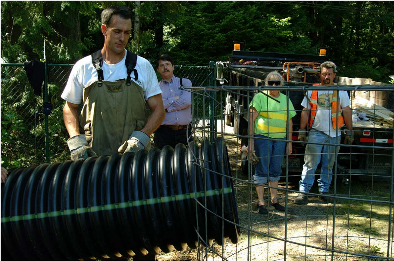
Inserting the pipe into the round fence filter.
