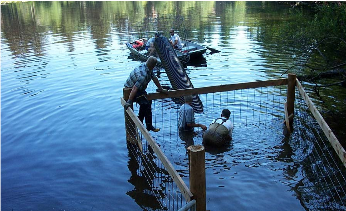
Peterson Pond dropped off to around 8 to 10 feet in depth shortly past the end of the receiver fence, a small boat was needed to move the round fence into place.
