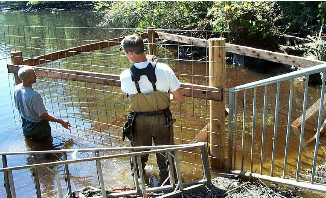
Attaching the fencing to the sides of the receiver fence.
