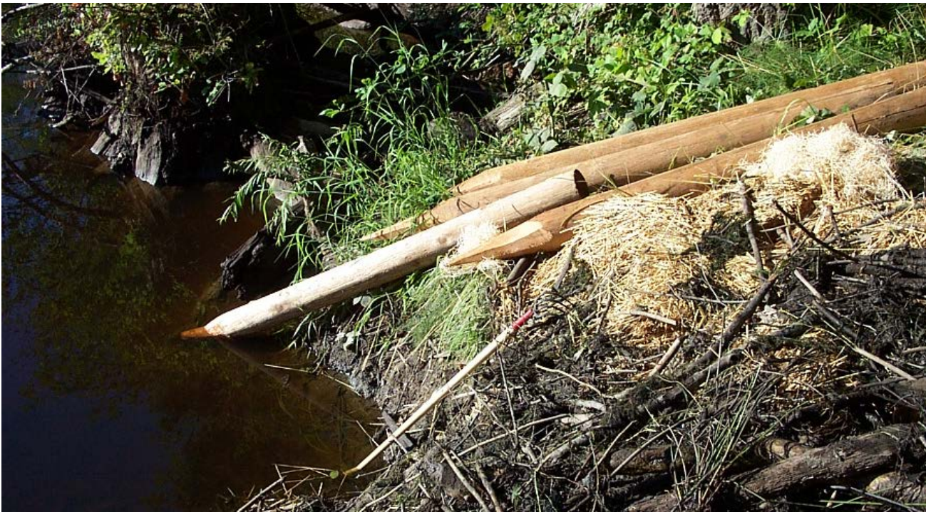
Sharpened corner posts at the water's edge.
