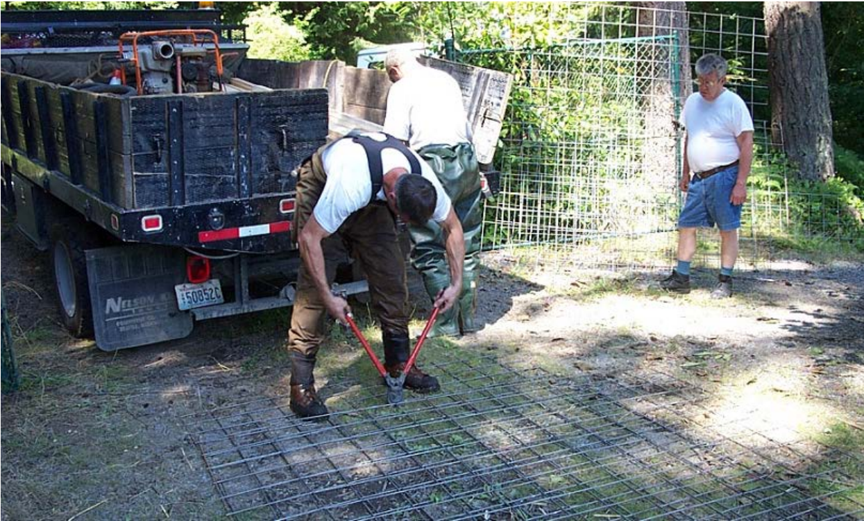
Cutting the fencing to match the contours of the pond bottom.
