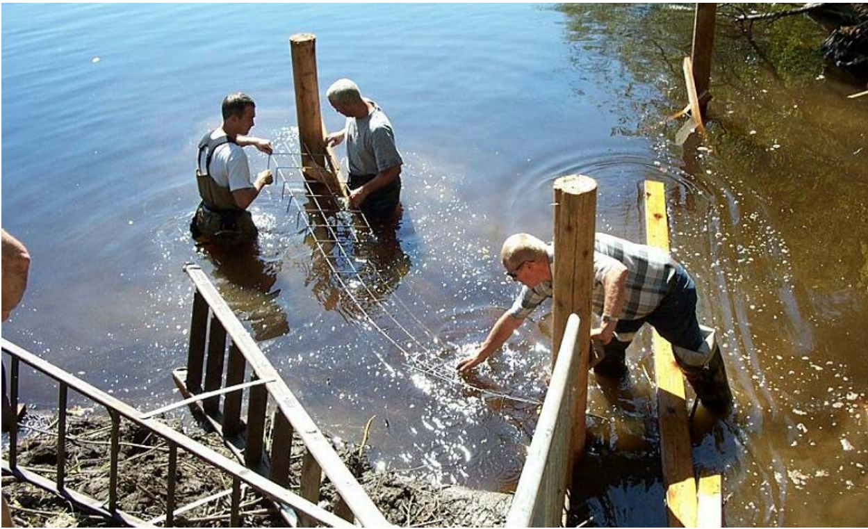
Installing the footing.
