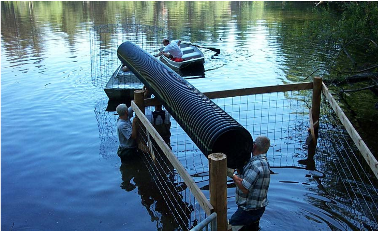
Moving the pipe into place by the receiver fence.
