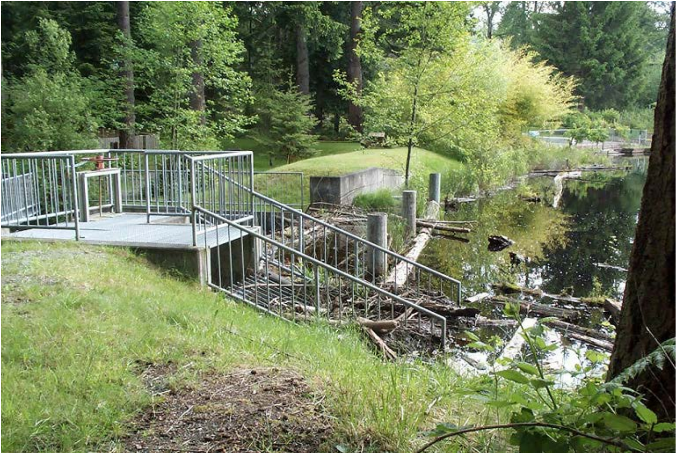
Trash rack blocked by beaver activity.
