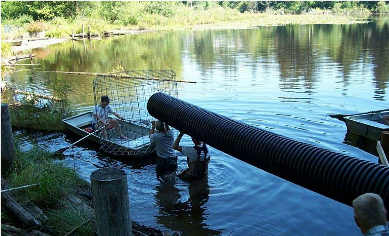
Moving the pipe and round fence out into position.
