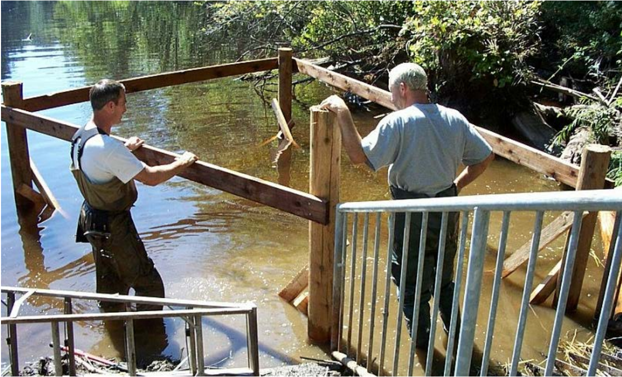
Attaching the stringers to the side posts.
